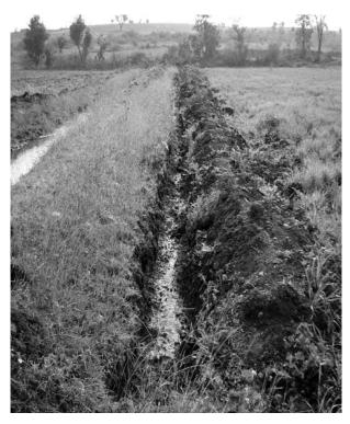
Fig. 16: Drainage Channels for Seepage
