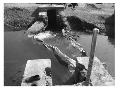
Fig. 17: Impromptu Bunds on the Main Canal Diverting of Water into Distributaries
