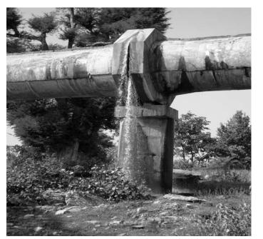
Fig. 9: Leaking Aqueduct
