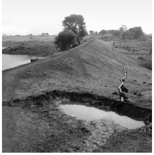
Fig. 12: Diverting Seepage Water for Irrigation
