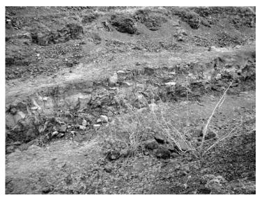
Fig. 8: Poorly Constructed Main Left Bank Canal
